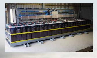
The remote site was installed with a 57kwp solar array which was ample to supply power to the business at all times, including nights and times with no sun. The off grid system was designed to store the excess power for these periods.
